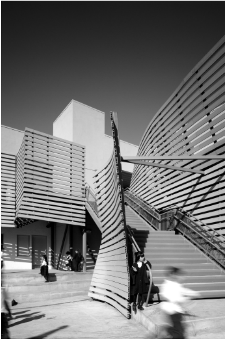
CNCA stair and courtyard
