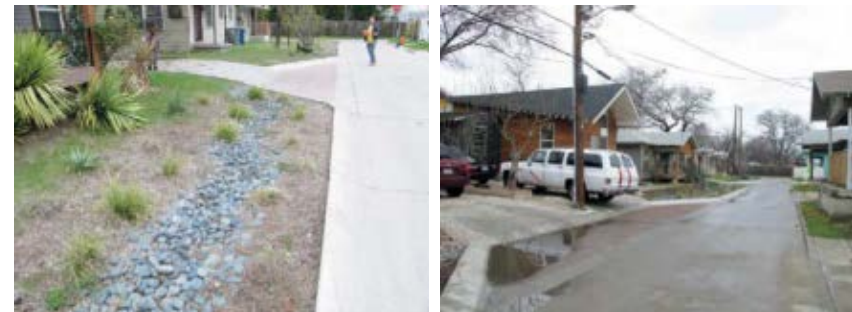
The reconstructed street includes permeable paving (with standing water at time of site visit) and a landscaped bio swale
