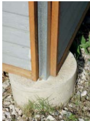
Planning meetings with residents and construction details
