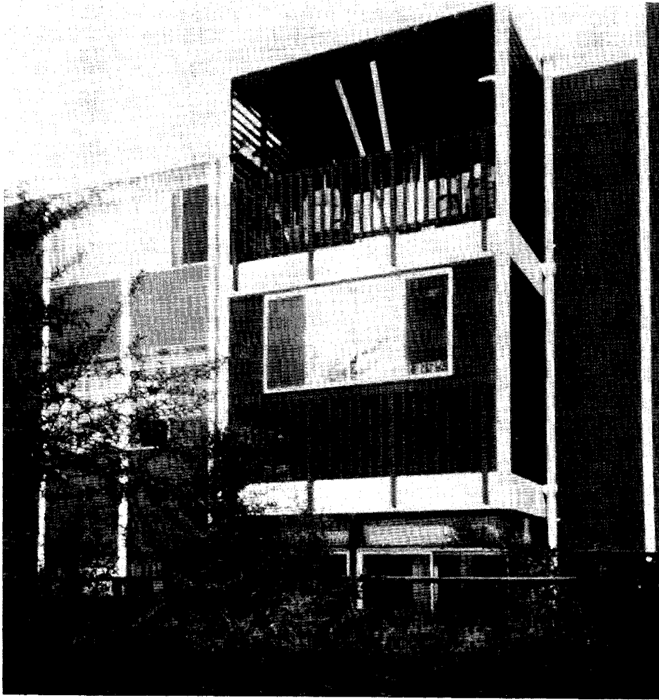
Fig. 3-12. Some residents have enclosed their balconies to gain additional interior living space.
