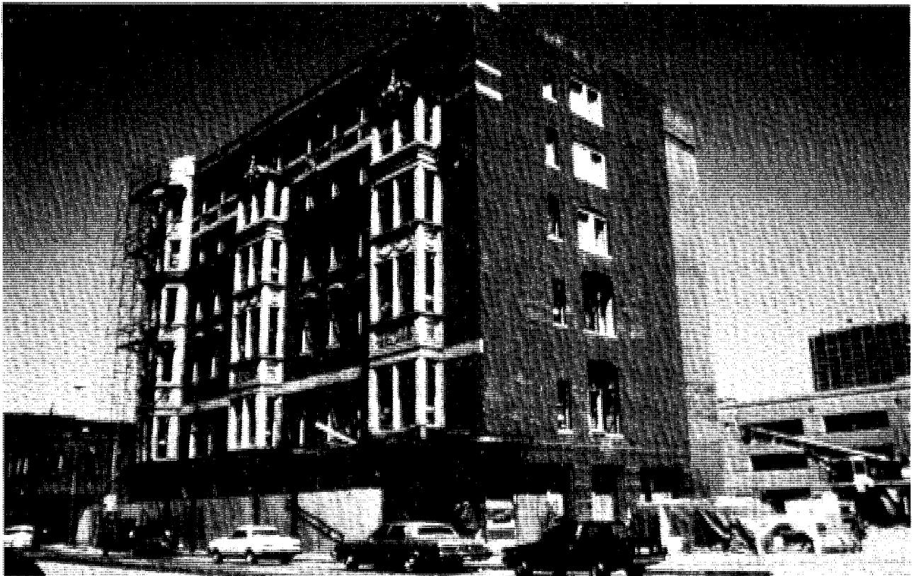
Fig. 4-7. The Coates House during restoration.
