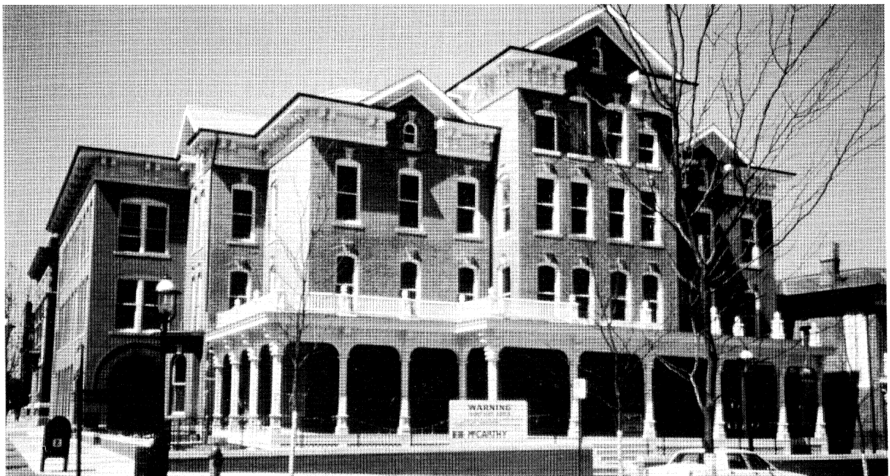
Fig. 4-11. The Virginia Hotel: today. (Courtesy of McCormack, Baron and Associates archives.)
