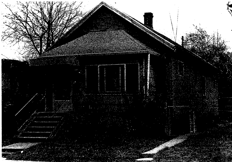
West Clinton home before renovation.
