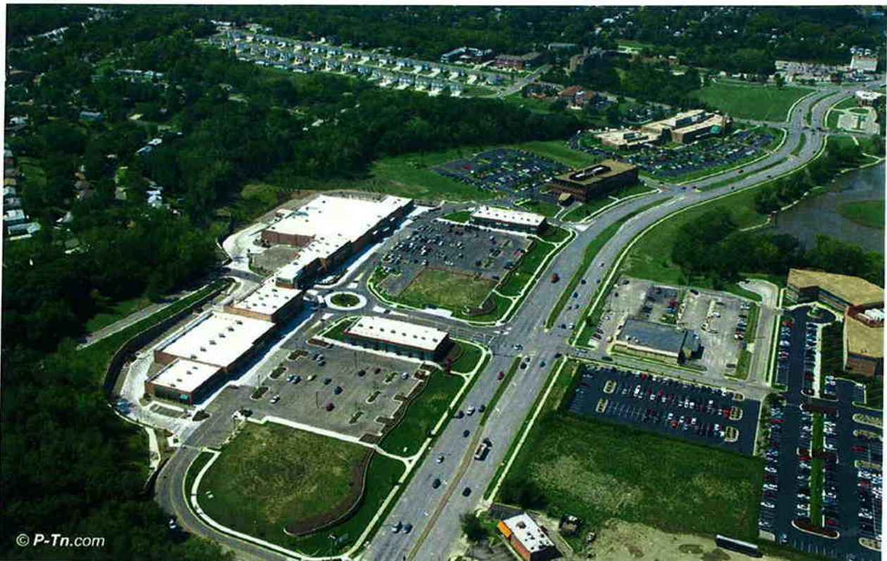
Blue Parkway Town Center – on right; H&R Block Building on left
