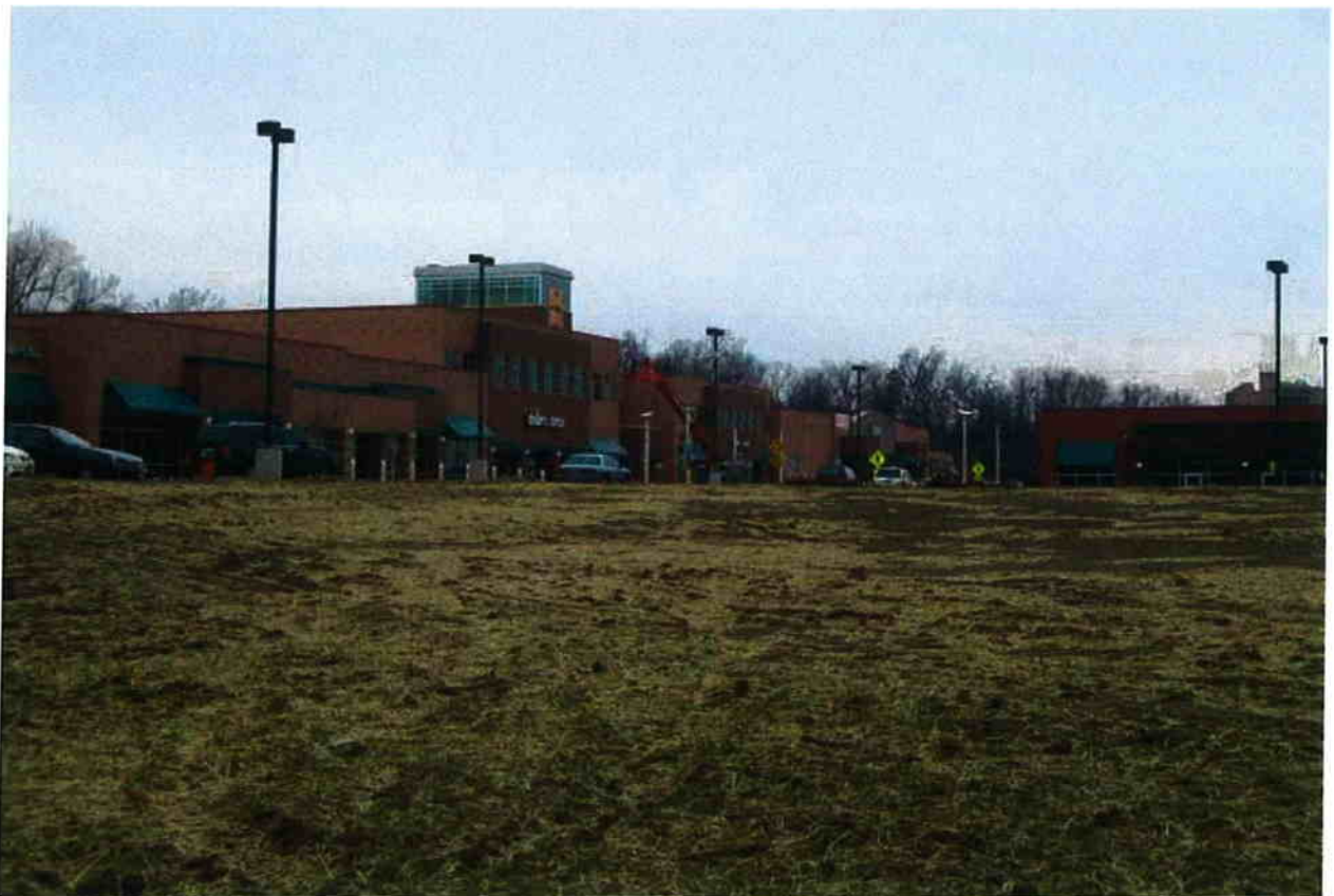
Blue Parkway Town Center under construction
