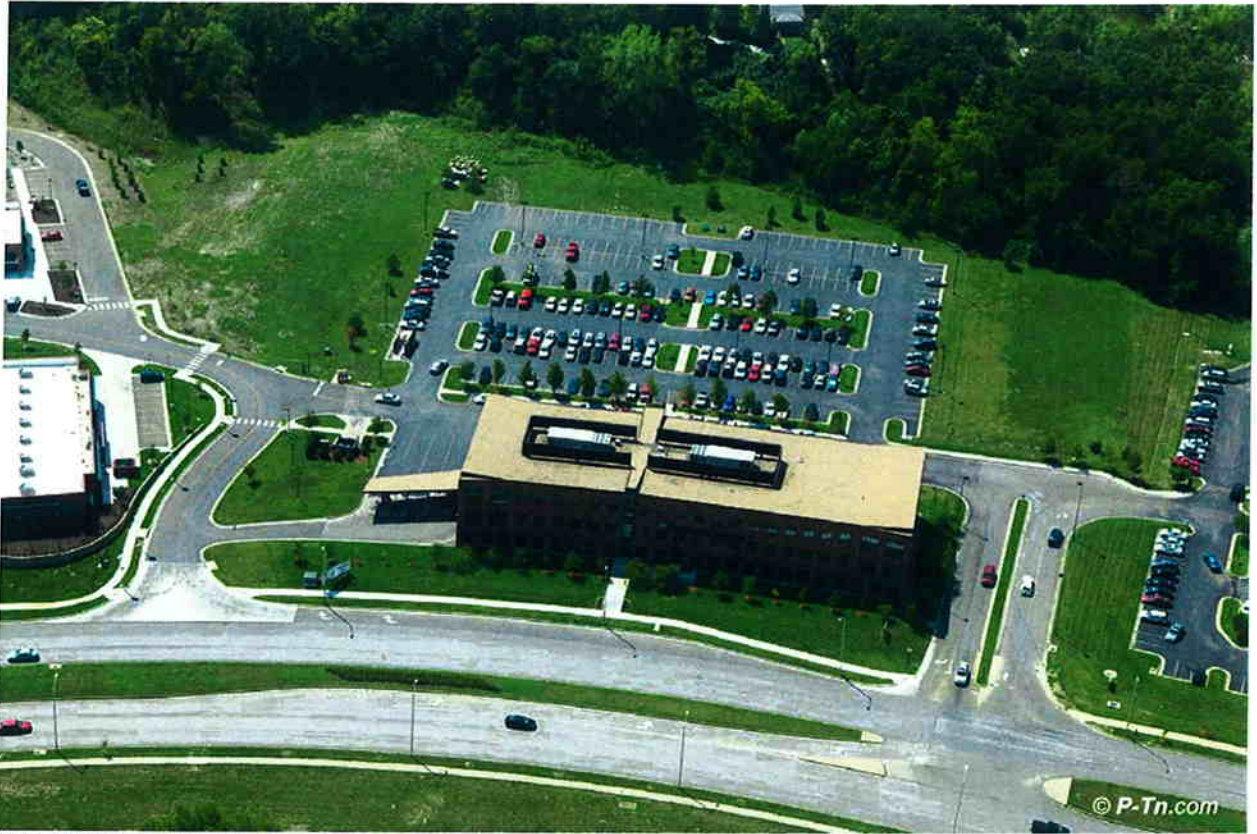
4001 Building – looking south across Blue Parkway
