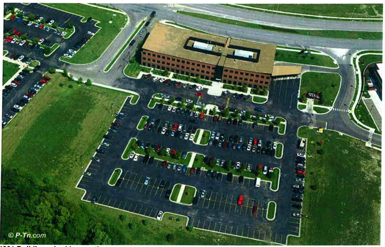
4001 Building – looking north
