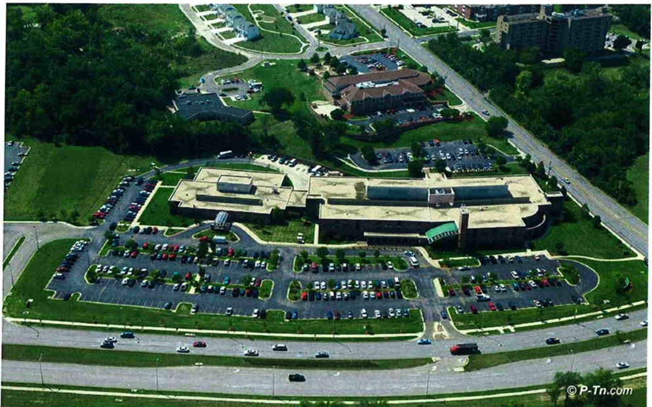
Swope Health Services – in foreground – looking south across Blue Parkway
