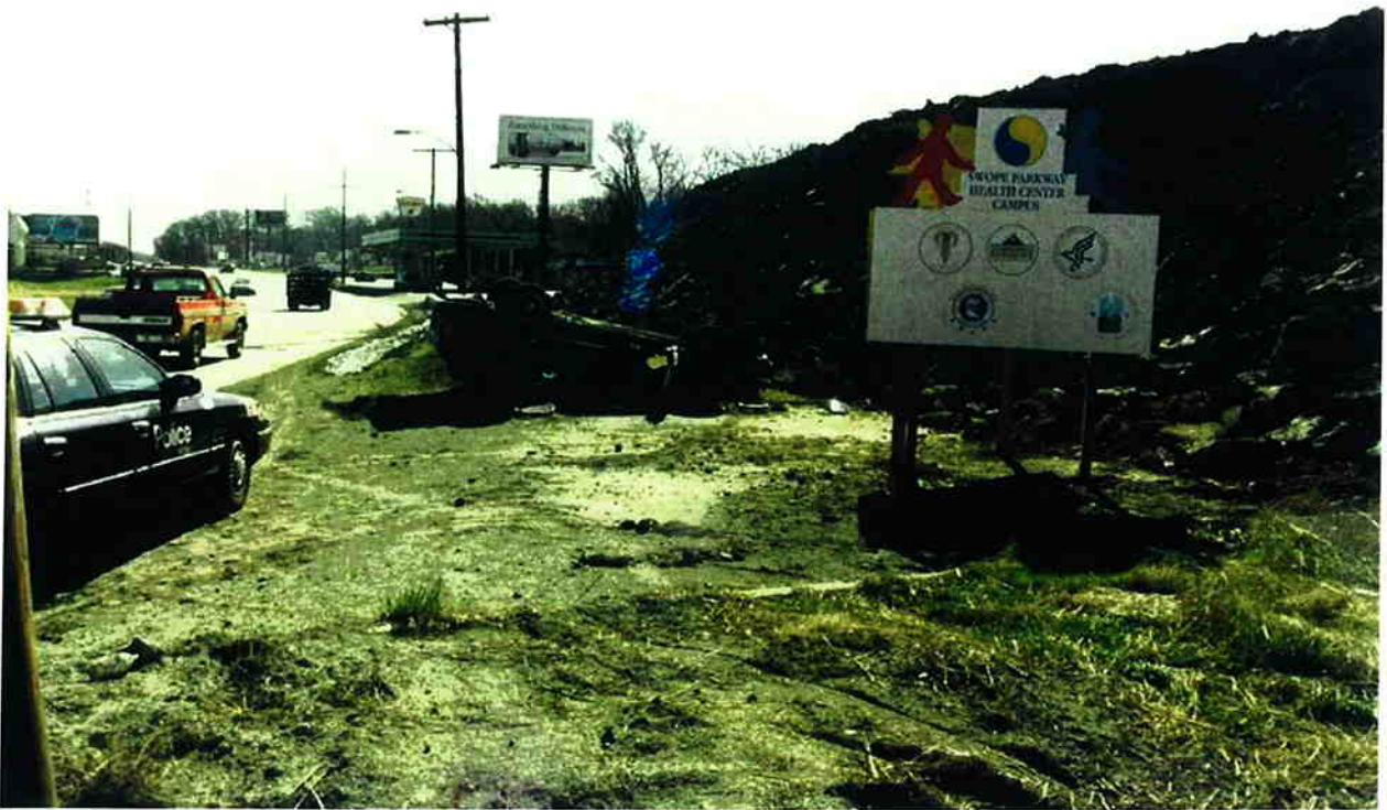
Site of Swope Health Center before construction – Note pile of land fill to raise site elevation
