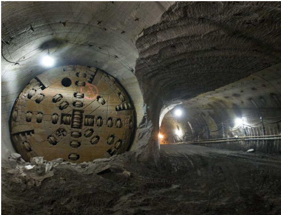
MTA East Side Access project
