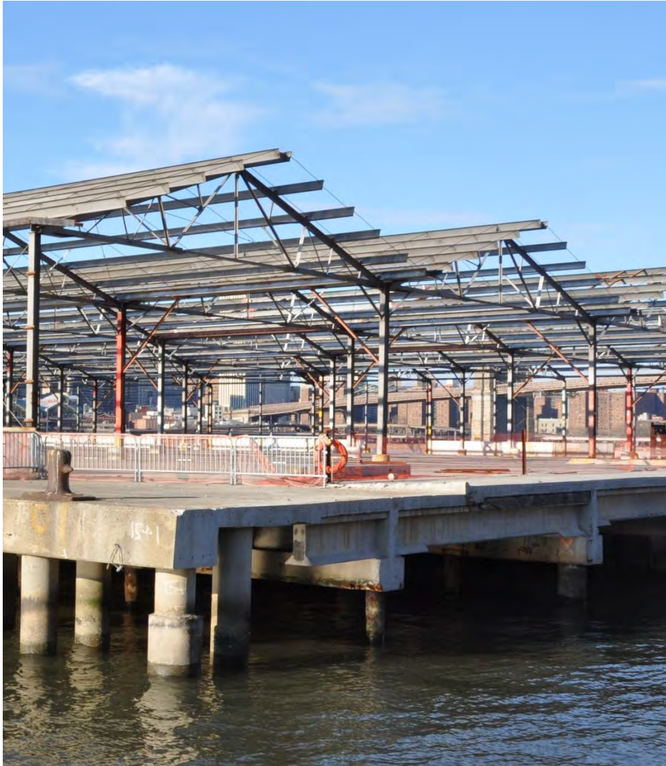
Pier 2 Shed Walls
