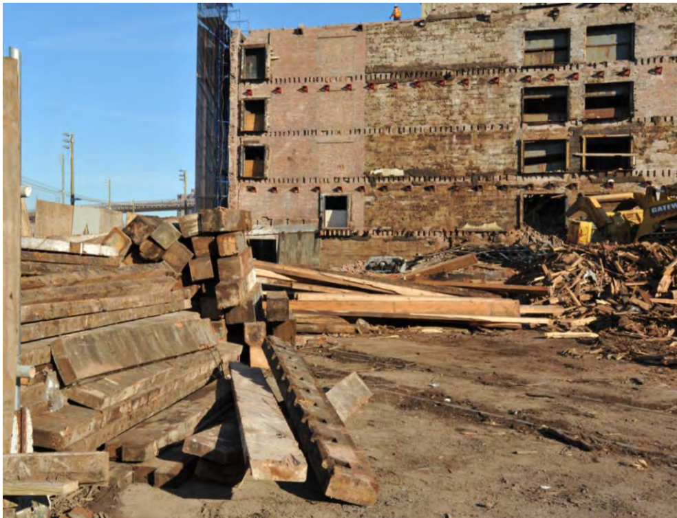
Cold Storage Warehouse Demolition
