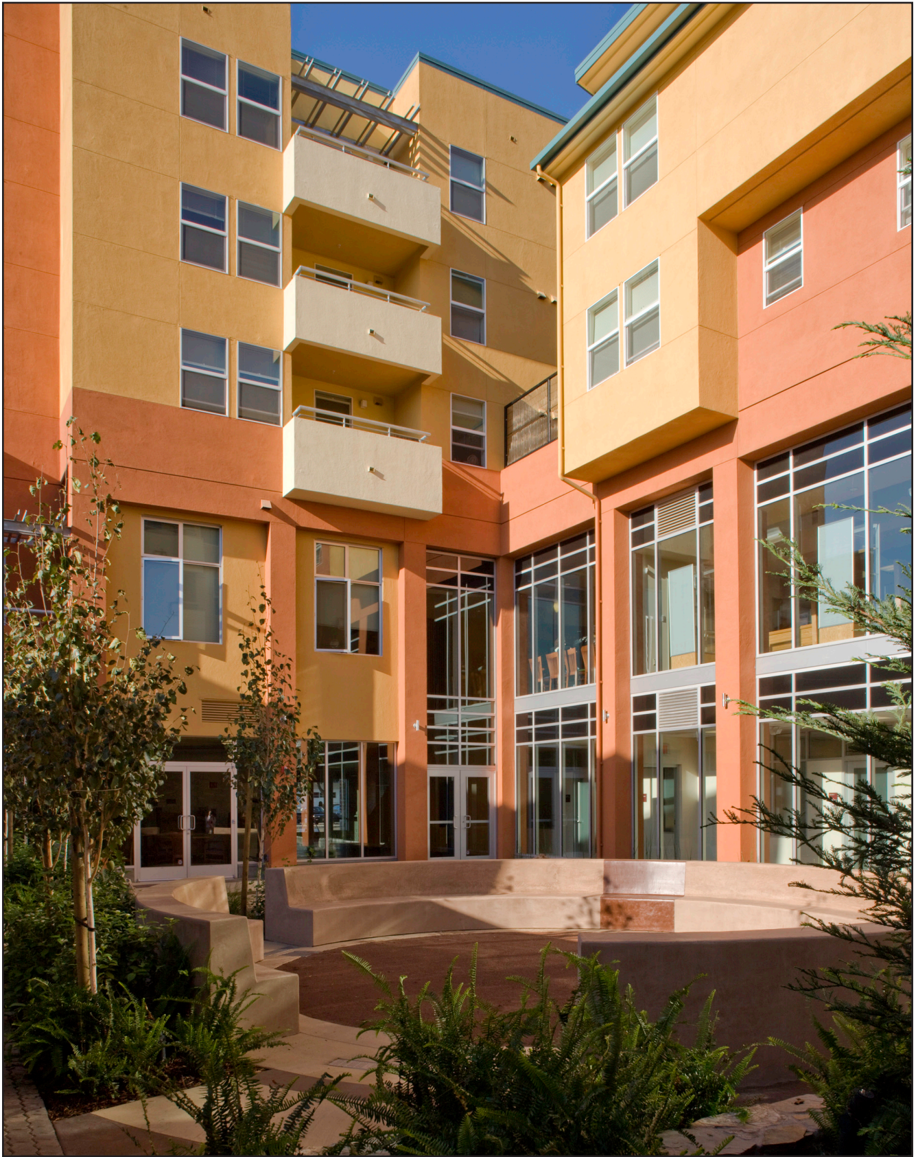
Clinic courtyard; second floor clinic gallery overlooks the courtyard and residential units above
