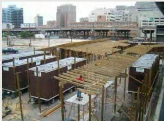
Construction of the Rebuild Center with trailers in foreground
