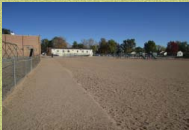
Existing condition of school yard includes 4 acres of pea gravel and 1950's play equip.
