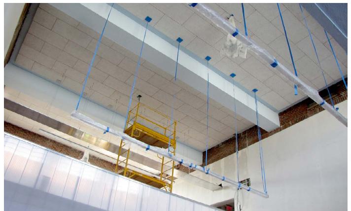
Overhead lighting installation in progress
