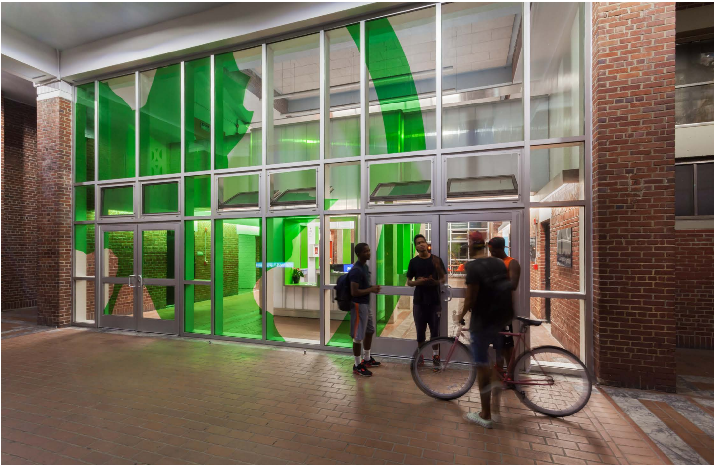
Completed storefront installation with NYCParks logo
