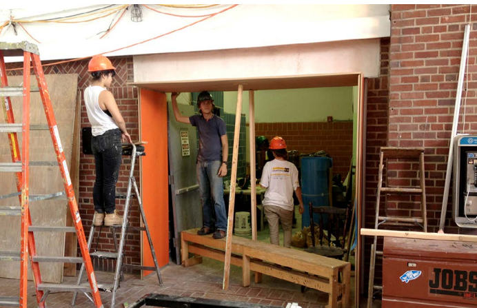
Installing pop-out threshold framing with lighting cove above
