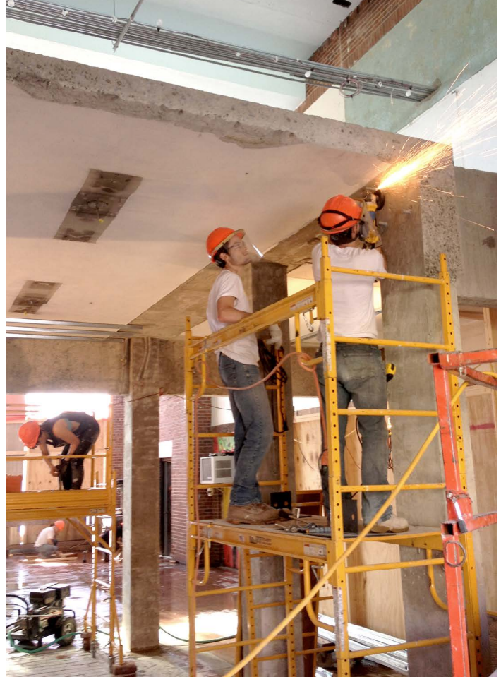
Installation of support structure for mezzanine level
