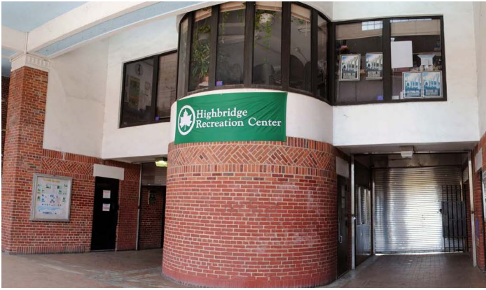
Main entryway prior to renovation
