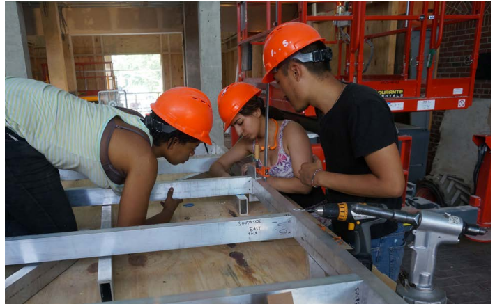
Constructing support structure for mezzanine level
