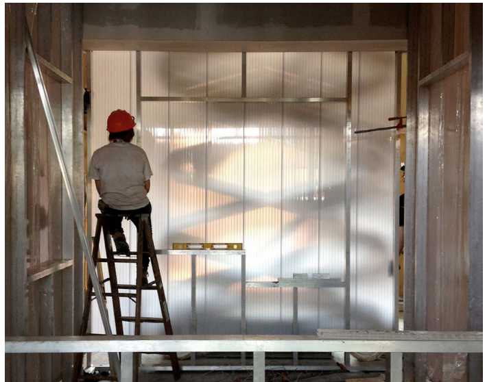
Installation of Duo-Gard sheeting around the reception desk
