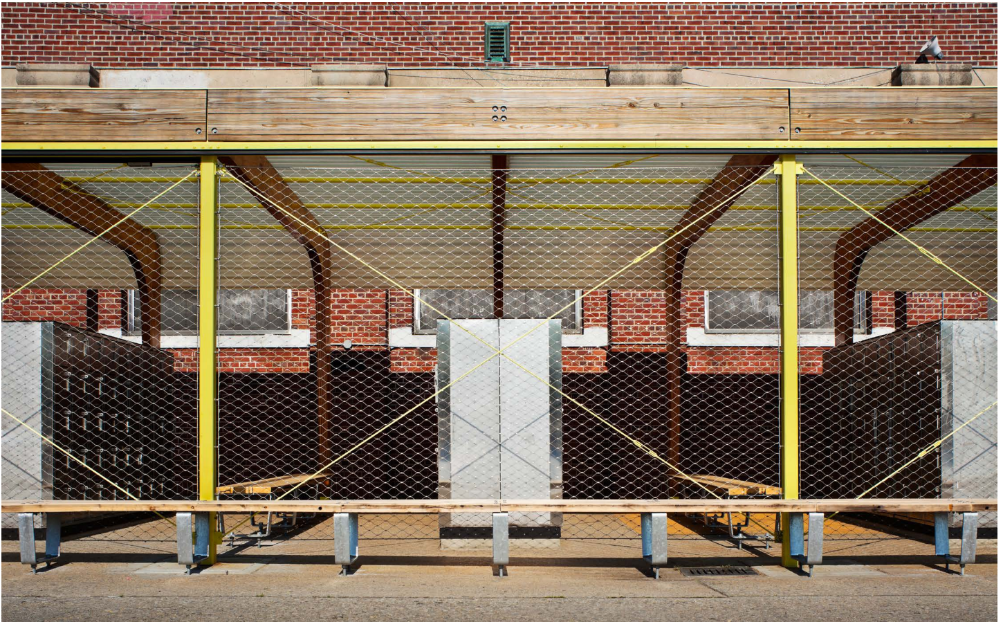
When the pool is at capacity, sliding doors can close off the locker room, creating additional changing rooms when in need.
