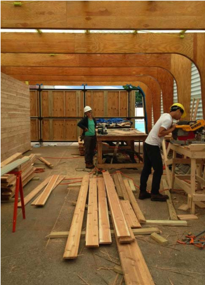
Cutting cedar cladding for exterior changing pavilions
