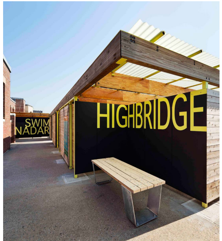
The structure is made from reclaimed cedar, plywood and translucent corrugation
