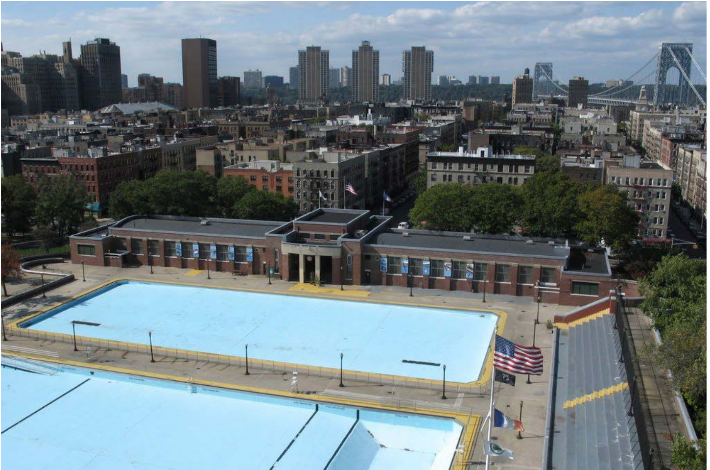
Center exterior prior to renovation. Aside from the addition of a breezeway in 1982, it had only received minor upgrades until the three-year partnership between Parsons and Parks began in 2011.
