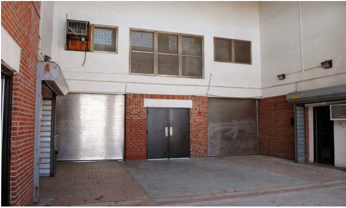
Interior breezeway prior to renovation
