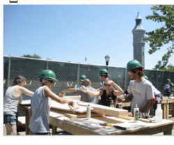
help drill the structure into place.
