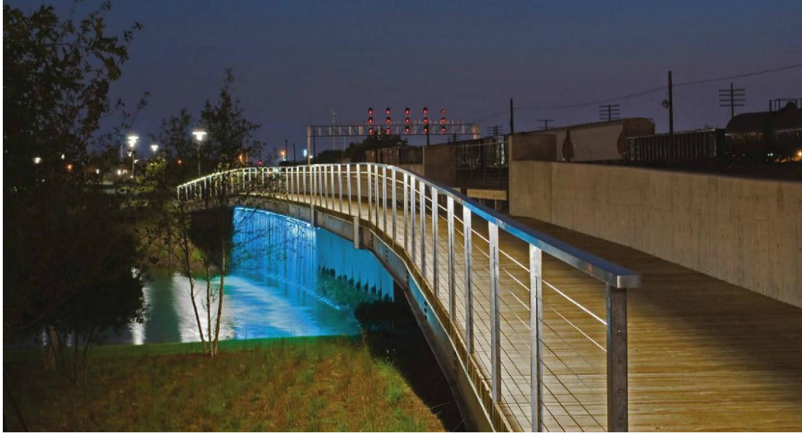
RR Park with Jogging Bridge and Rain Curtain at Pond Parallel to Train Tracks
