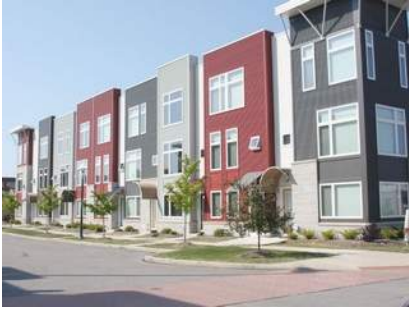
New townhouses in Cleveland's Battery Park redevelopment project, which used city tax abatements.
