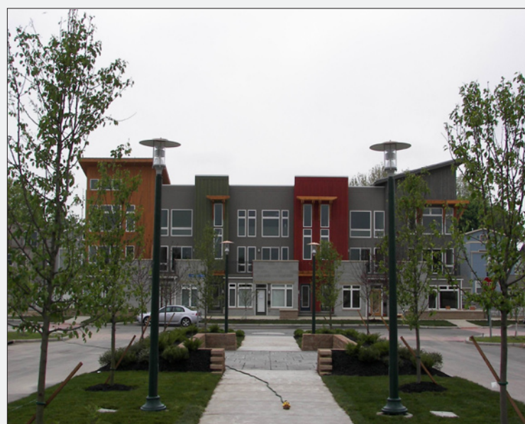
THE 'AVENUE BUILDINGS' WERE SEVERAL OF THE FIRST TO BE BUILT AT BATTERY PARK.
