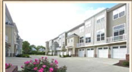
Courtland Court Project -Mike DeCesare
