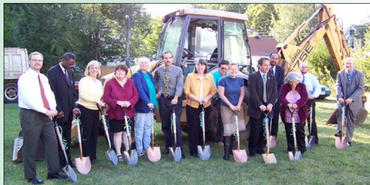
September 9, 2008 Green Cottages Groundbreaking: Digging the ceremonial first shovel are (left to right): Jim Ptacek, Eddy Chatmon, Betsy Figgie, Beverly Jones, Dolores Watson, Piet Van Lier, Marge Misak, Dave Fragapane, Mandy Metcalf, Councilman Matt Zone, Daryl Rush, Ruby Collins, Matt Wooten, and Jeff Ramsay
