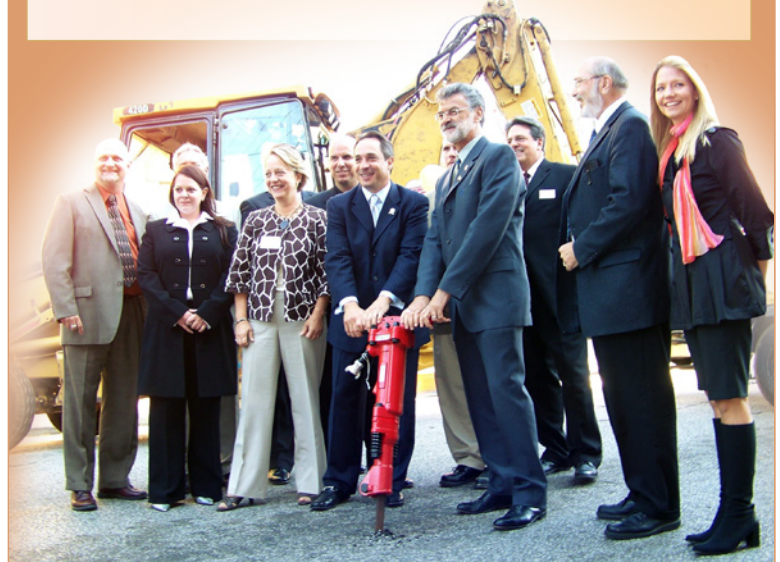
DETROIT AVENUE STREETScape CONSTRUCTION HAS BEGUN. HOLDING THE JACKHAMMER AT THE GROUND-BREAKING CEREMONY ARE MAYOR FRANK JACKSON AND COUNCILMAN MATT ZONE.
