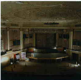
Current state of the interior as we get ready for construction
