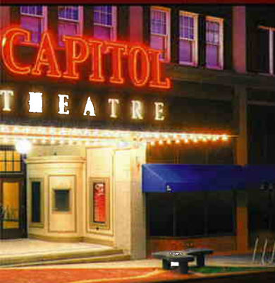
photo: Marous Bros. Construction
