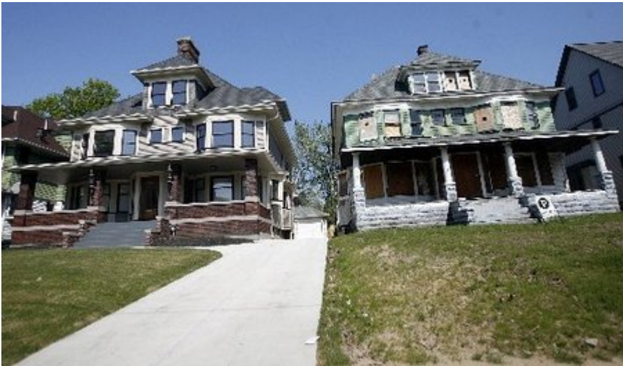
MICHAEL DeMOCKER / THE TIMES-PICAYUNEA boarded-up house in the University Circle neighborhood stands side by side with a newly renovated home.
