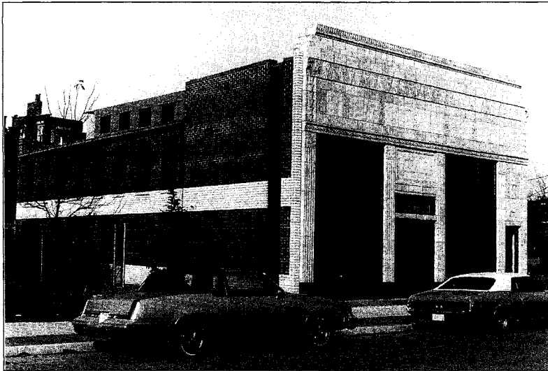
Preservation of historic facade with new building
