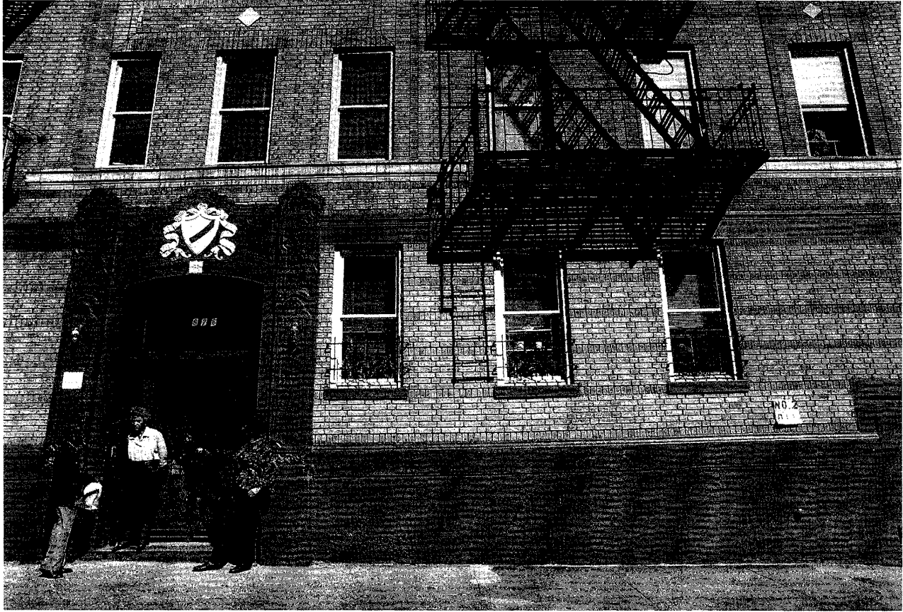
Hope is very much alive at 676 St. Nicholas Avenue. For the tenants who worked to restore the building, co-ops cost $250. (Photograph courtesy of Hazel Hankin, Brooklyn, New York)
