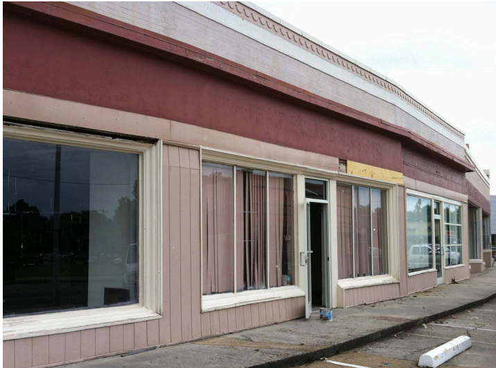
Crosstown Arts moved into a vacant storefront space across the street from the development site.
