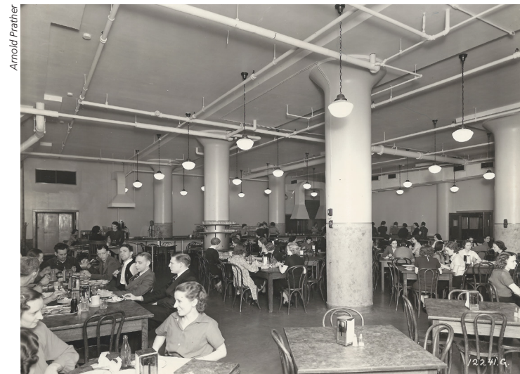
The building followed a standardized design that used a grid of reinforced concrete piers.
