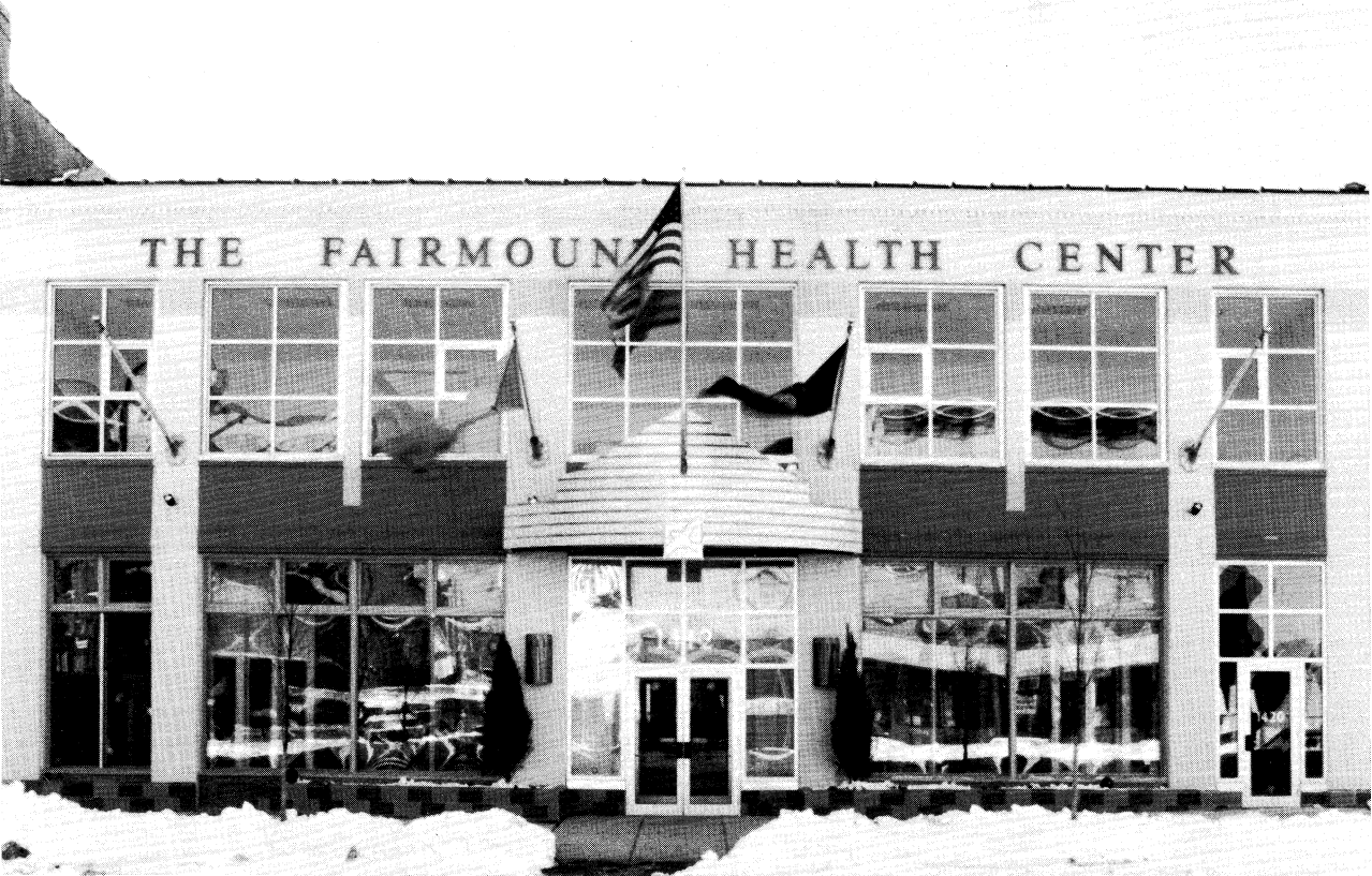
Fig. 6-8. The renovation completed. (Courtesy of Dagit Saylor Architects.)
